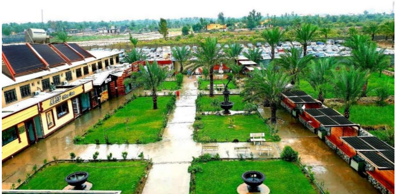
Figure 1. Use the solar water heater on the roof of the shopping book center
